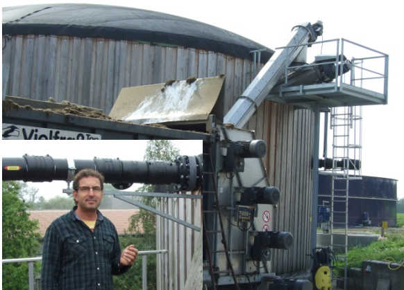
Figure 18: A biogas plant from a general contractor does the job at the organic Krumberger Hof of farm manager Gerhard Moser (small photo). Photos: F. Gerlach, FiBL.
