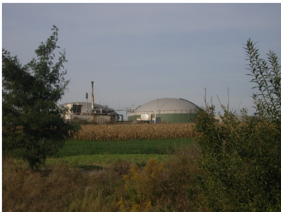
Figure 9: The largest dairy farm in Spain operates one of only 32 agricultural biogas plants in the country with slurry from 2,500 cows. The digestate is dried and sold as fertiliser for organic agriculture. Photo: STUDIA.
