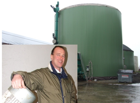
Figure 17: Hubert Miller, organic crop farmer in Schmiechen/Germany since the 1980s, has been running a 350 kW biogas plant with extra high fermenter and vertical stirring for six years. He uses a substrate mix with up to 98 % clover grass from about 40 organic farms. Photo: F. Gerlach, MEP.
