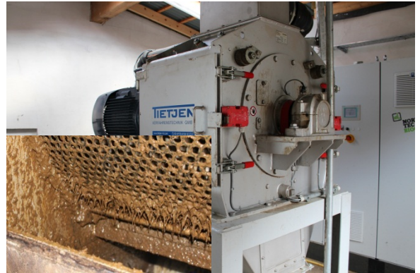
Figure 22: For medium sized and large biogas plants, disintegration techniques like this combination of hammer mill and specific microorganisms, can improve efficiency and reliability. Photo: F. Gerlach, FiBL.
