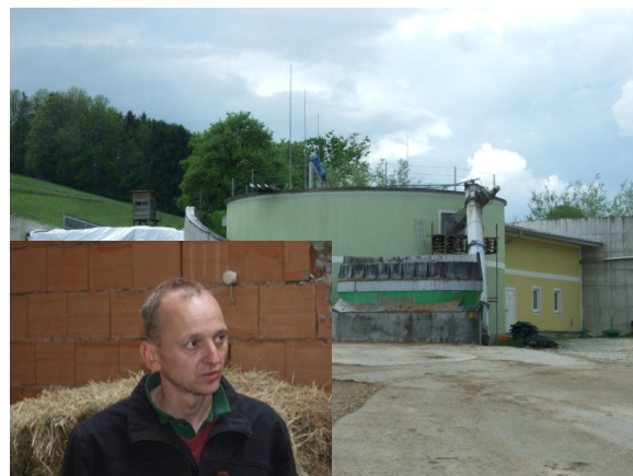
Figure 8: Gerhard Übleis operates a biogas plant in Schwanenstadt/Upper Austria with a mix of organic and conventional input. The heat is used for drying wood chips as fuel. Photo: F. Gerlach, FiBL.
